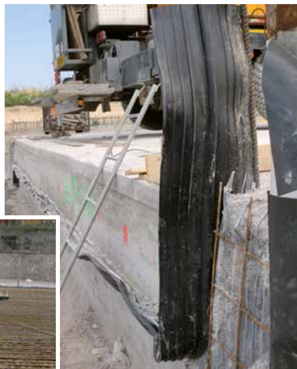
Application du joint WATERSTOP BFO
